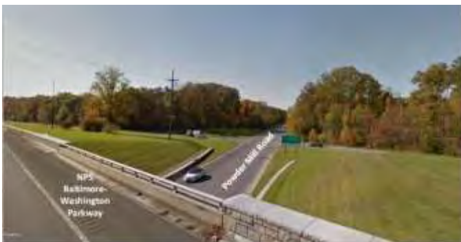
View from BW Parkway onto Powder Mill Road.
