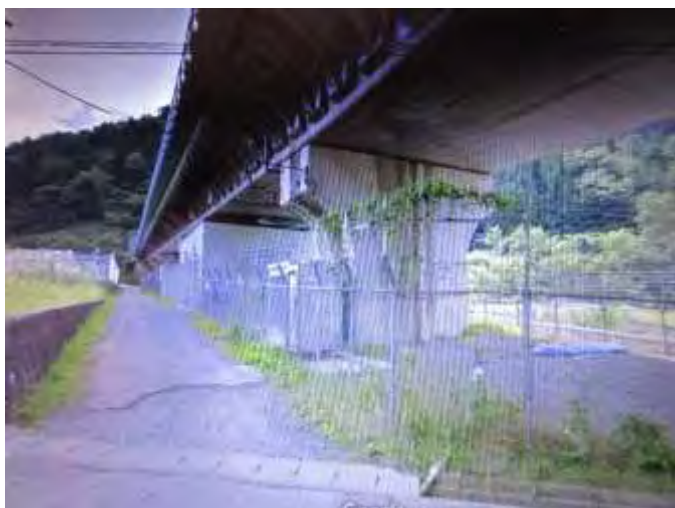
Reality - SCMagLev viaduct fencing in Japan - photo 1.
